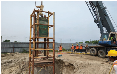
Pile Driving Analyzer (PDA)
