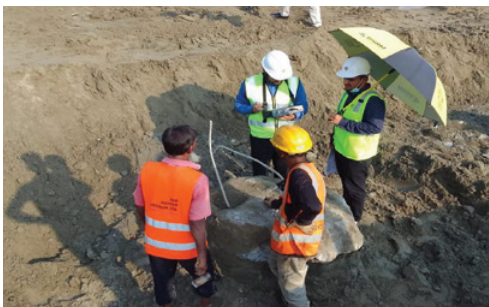
Pile Integrity Test (PIT)
